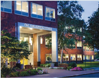
Burlington Woods Office Park, Burlington MA
